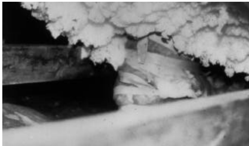
A condensation and freezing nightmare, ice hangs from the underside of the roof deck in this attic.
