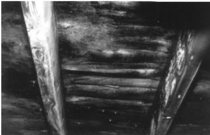
A roof deck and rafters darkened by rot show that this attic has severe moisture problems.
